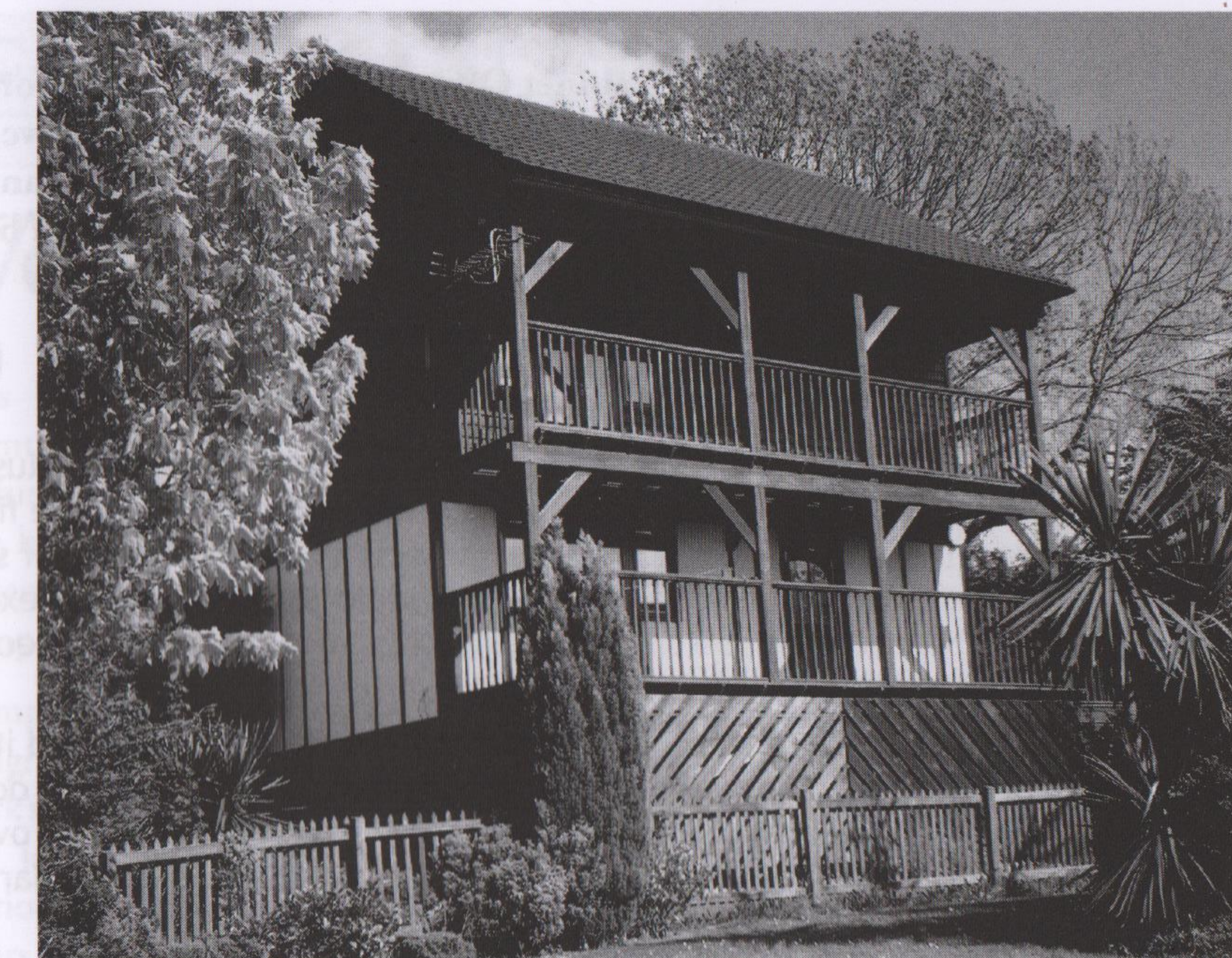
One of the self-built Walter Segal houses at South Petherton completed in 1996. South Somerset District Council initiated the scheme and sold the land to Knightstone Housing Association for £1. The project took over three and a half years to go through planning, and just 18 months to build. Mr and Mrs X, one of the families participating in the scheme, were supposed to get £50,000 sweat equity in their home, but by the time everything had been paid for there was only £5,000 which they opted to spend on fittings. Thus they have ended up as tenants of the Housing Association, paying more than they would in a council house for the house they built. They are very pleased with the house — "you look after it more if you built it yourself" — but not at all pleased with Knightstone, whom they accuse of overcharging and "moving the goalposts".
