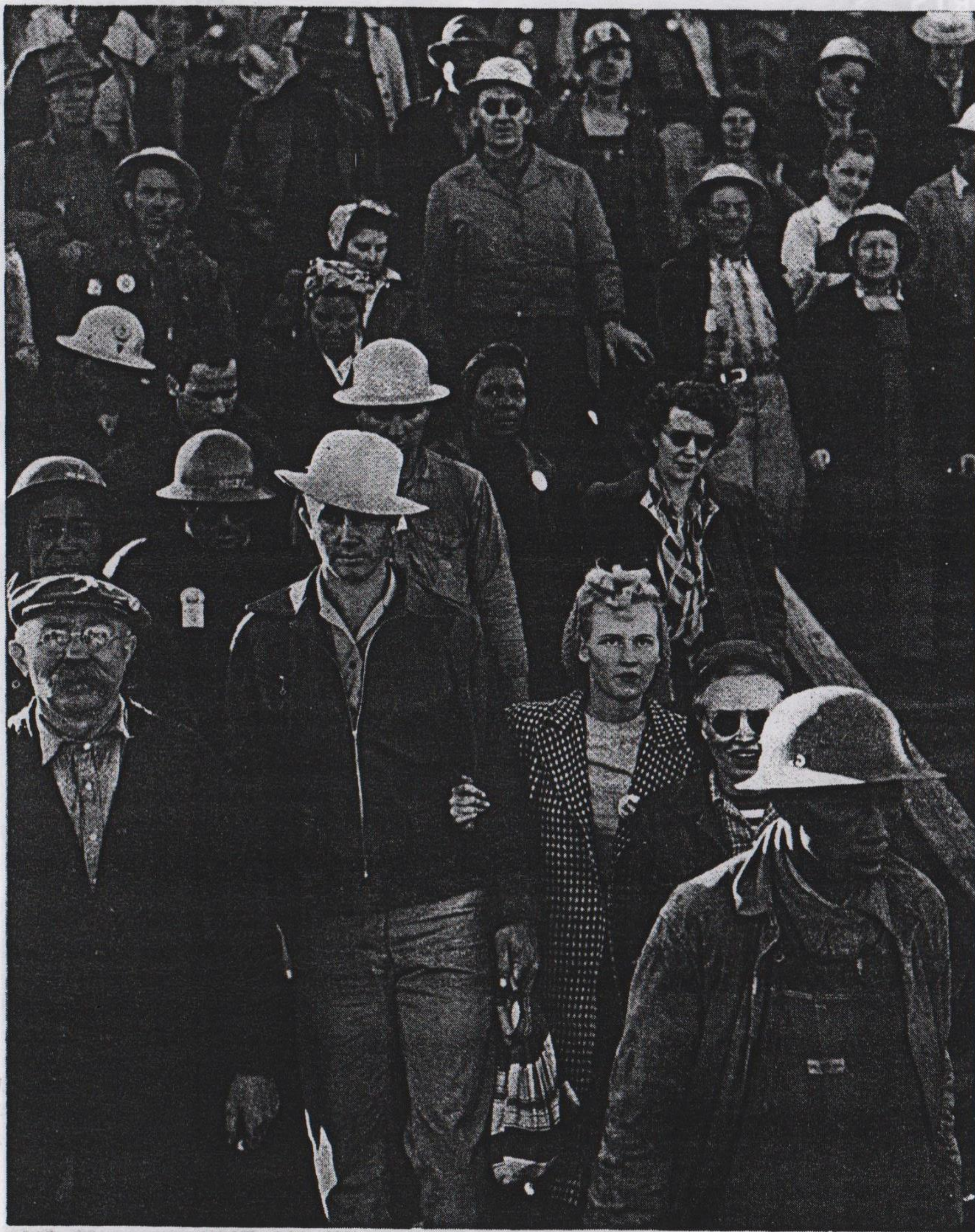
—Shipyard Construction Workers, Richmond, California.
