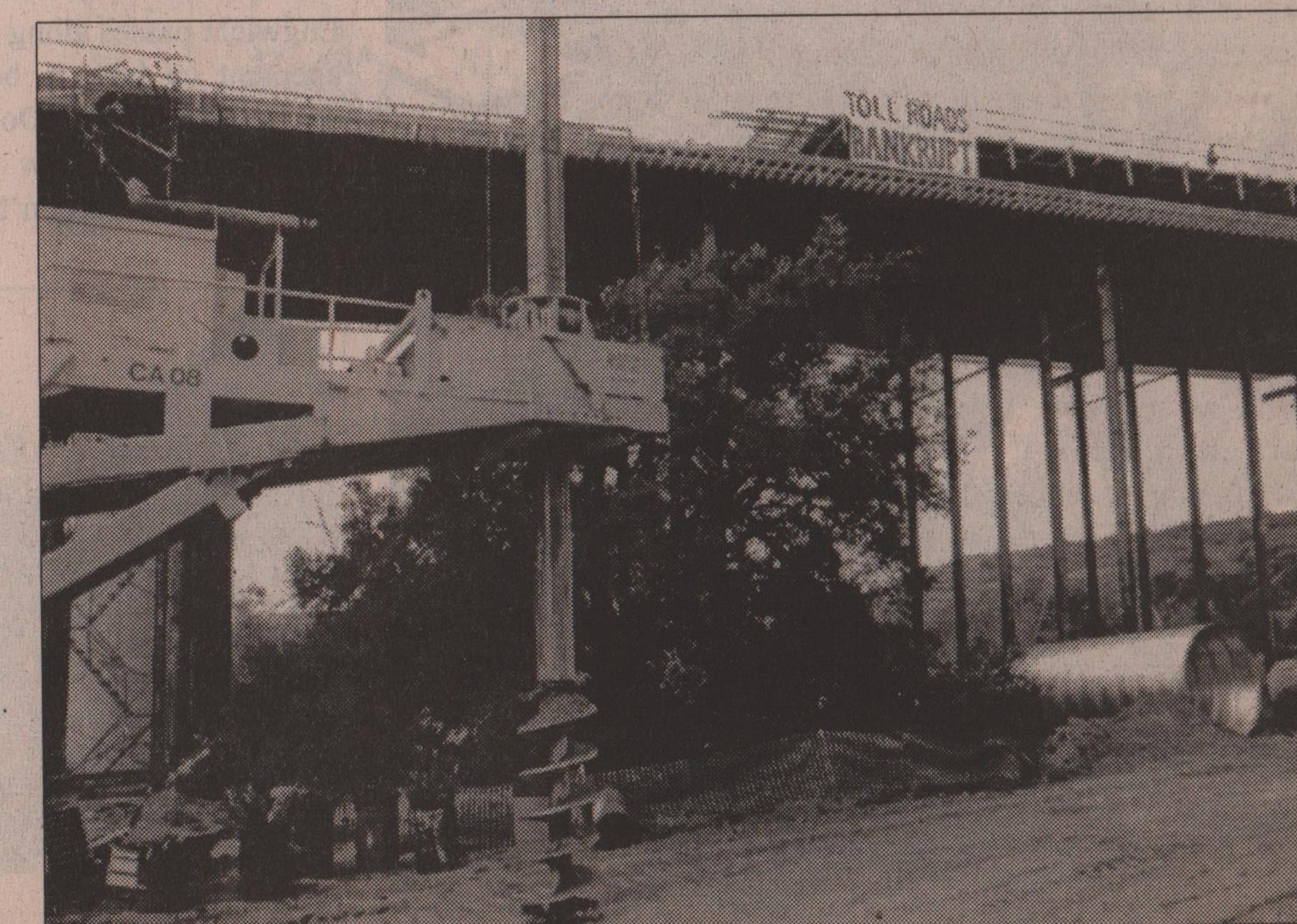
Foothill Tollroad construction site, February 8th, 1994. Day long Earth First! action. Photo by Randy Ghent
