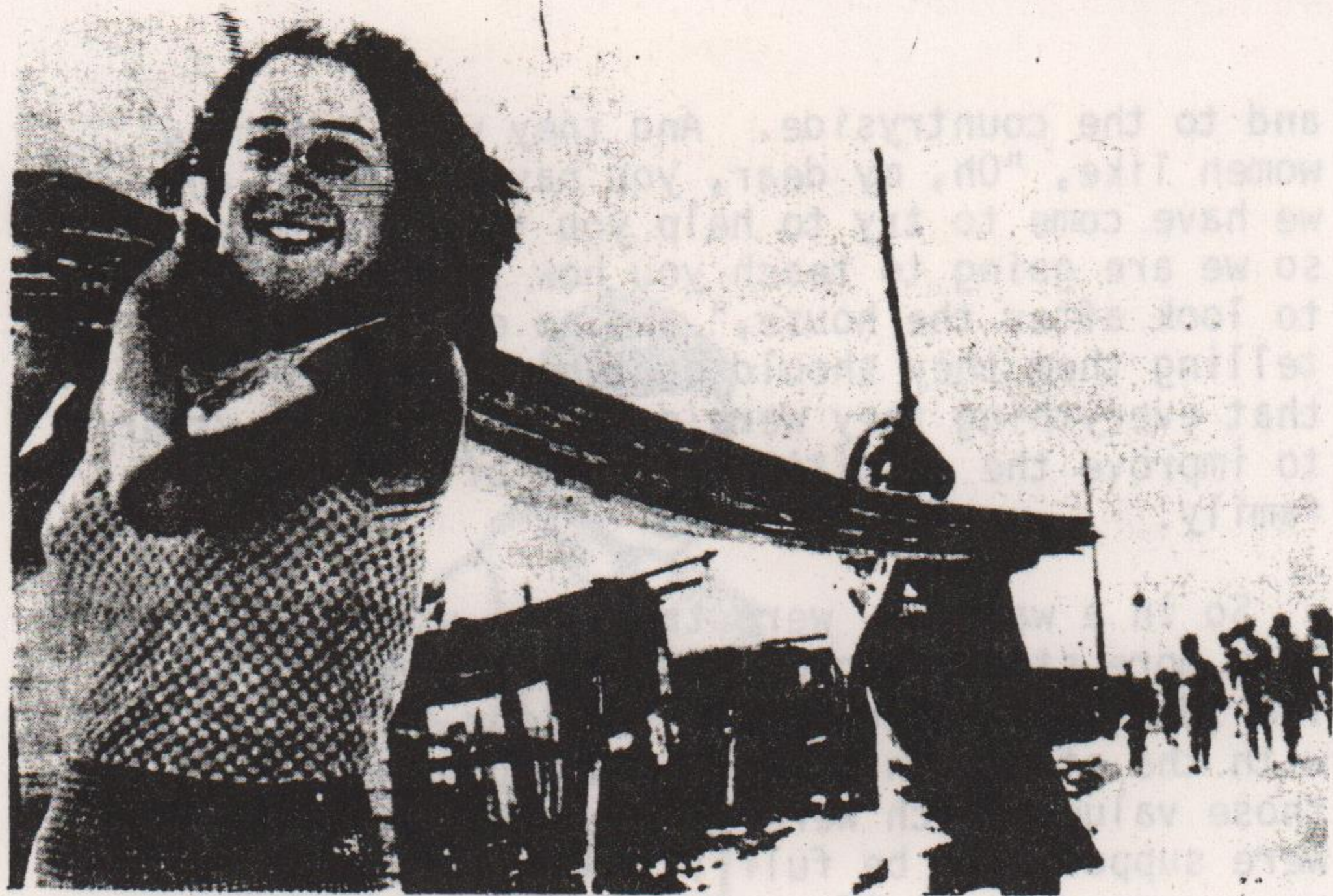
Building a campamento
