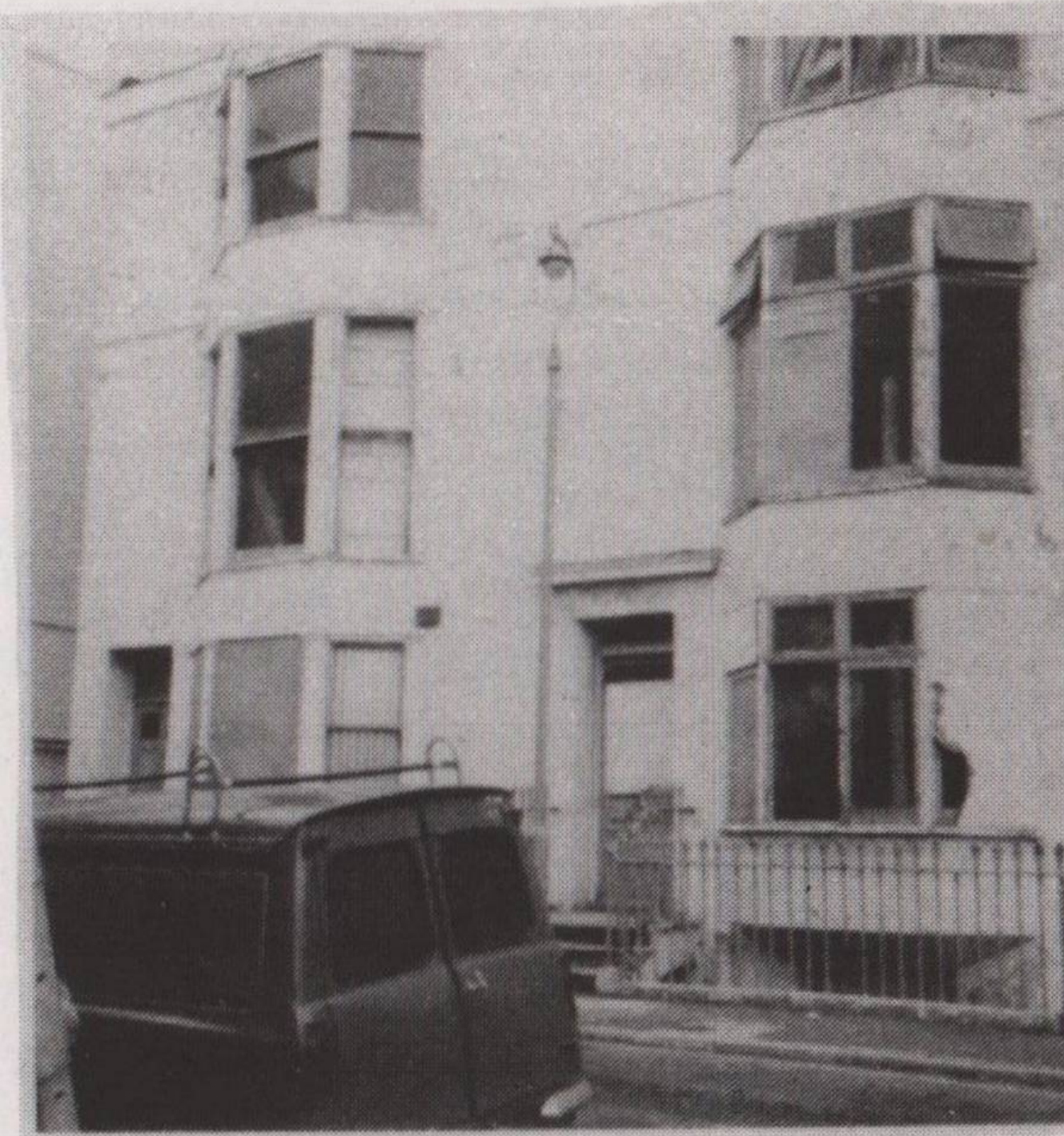
THE HOUSES IN RUSSELL SQUARE THAT BRIGHTON COUNCIL HAVE ALLOWED TO ROT - RATHER THAN LETTING THE CO-OP RENOVATE THEM TO HELP HOUSE THE HOMELESS.
