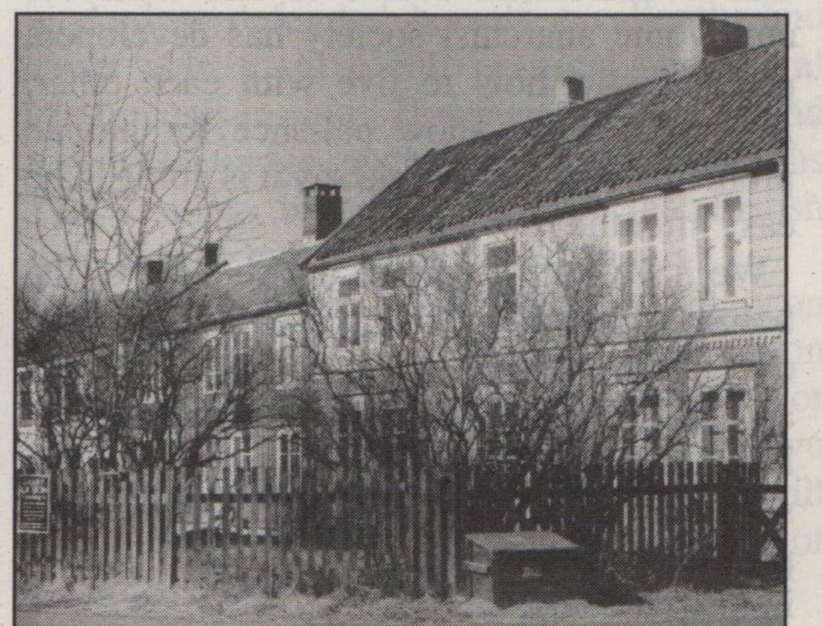
These small working-class houses from the 1870s are heavily threatened. (Photo: Oddgeir Havan)
