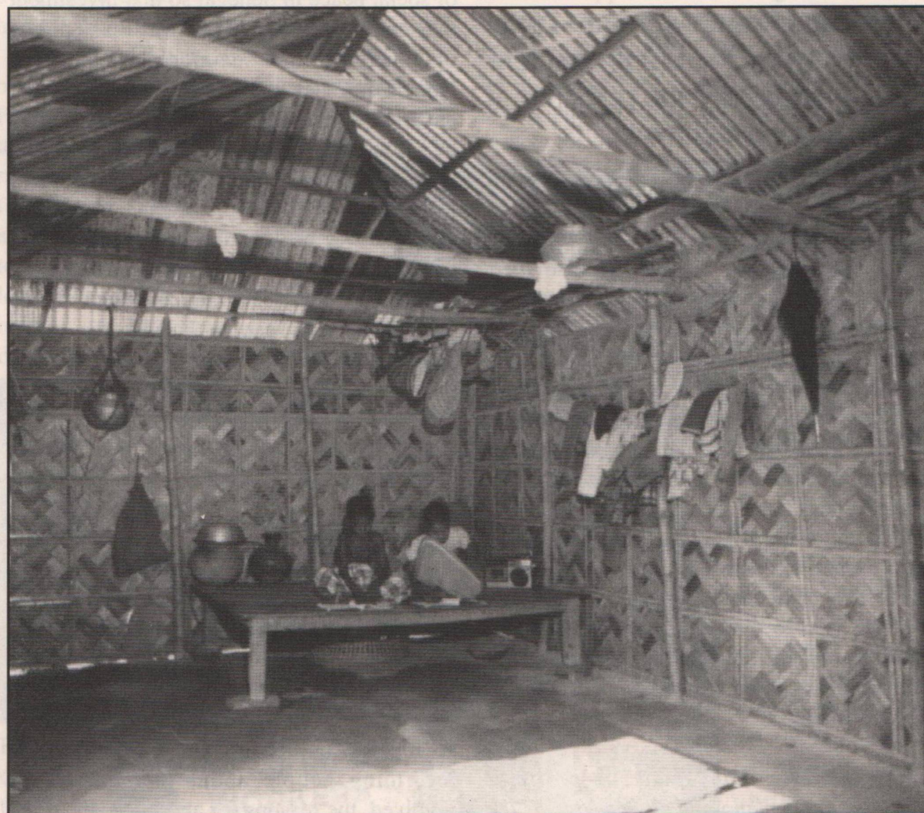
A rural Bangladeshi house. The concrete corner posts and roof sheeting are funded by the Grameen Bank and will survive floods. The bamboo walls are made by the family. When the floods come, the family will climb on the roof and will sling their belongings from the roof trusses.
