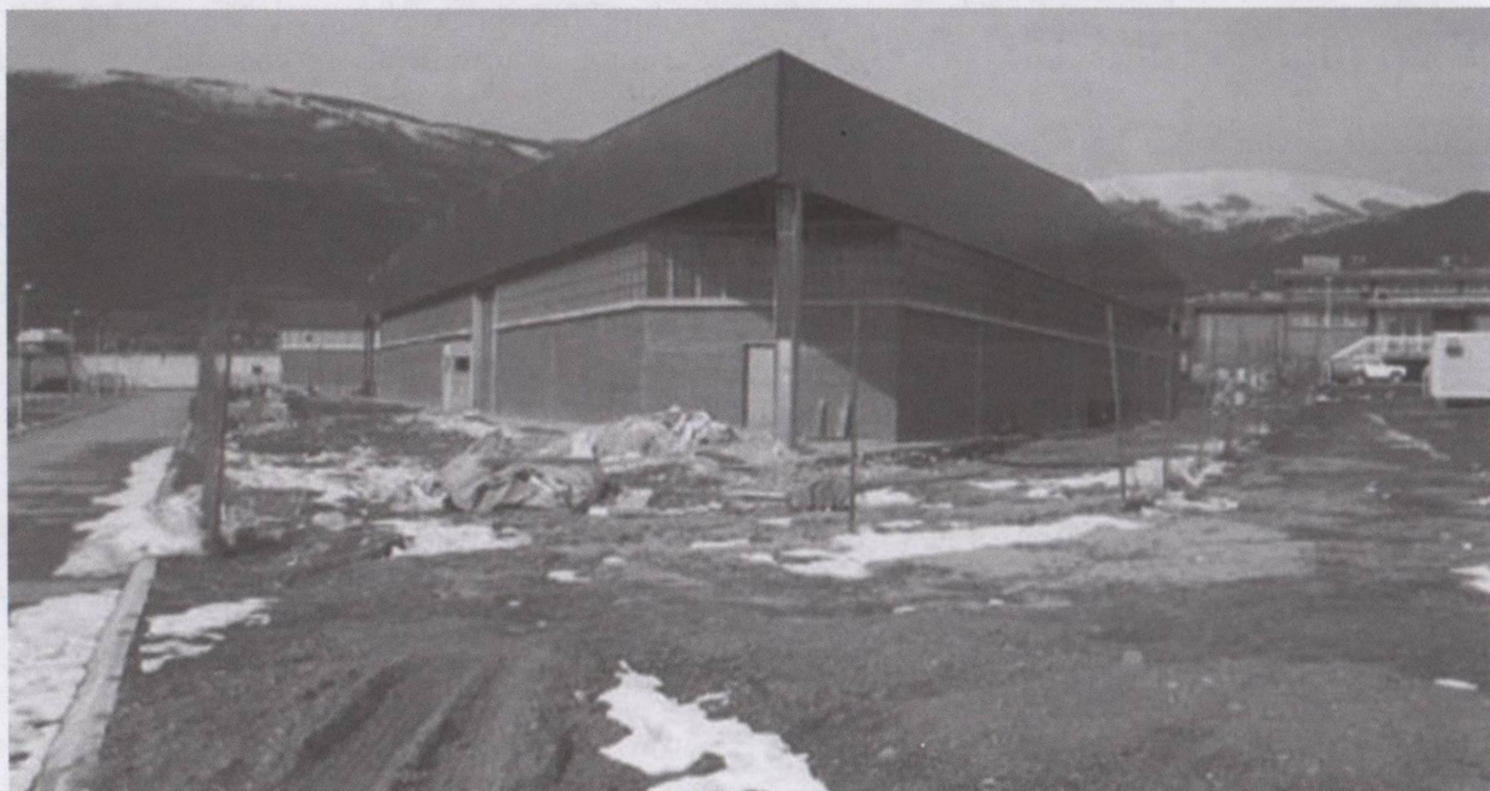
REBUILDING: Workshop 2 at Dubrava prison
