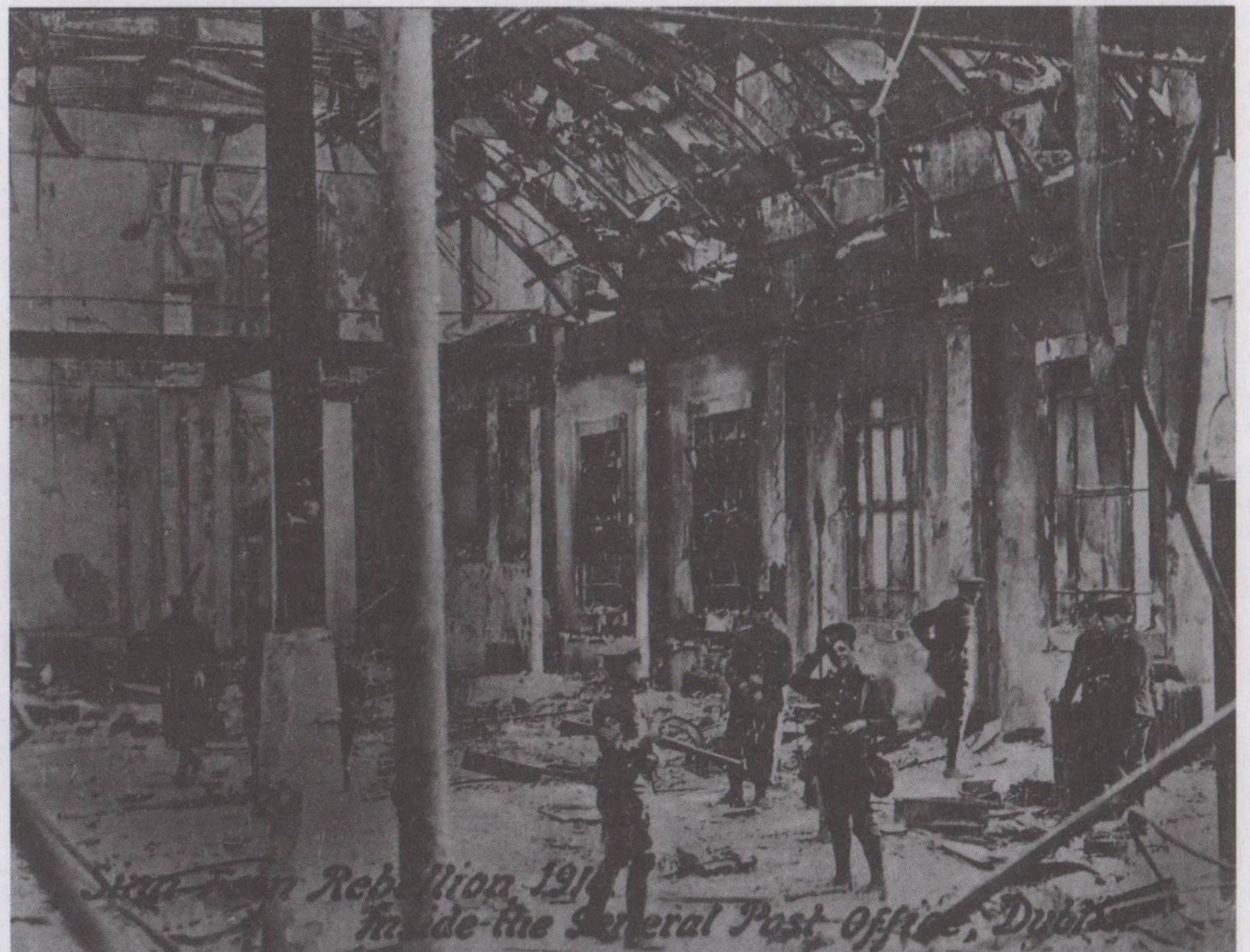
In 1916 Padraig Pearse and James Connolly, leaders of the Easter Rising, proclaimed an Irish republic from the steps of Dublin's post office. In the ensuing siege, the republicans sheltered and fought from within the building. A fire broke out, destroying most of the interior, and the post office remained closed for renovations until 1929.
