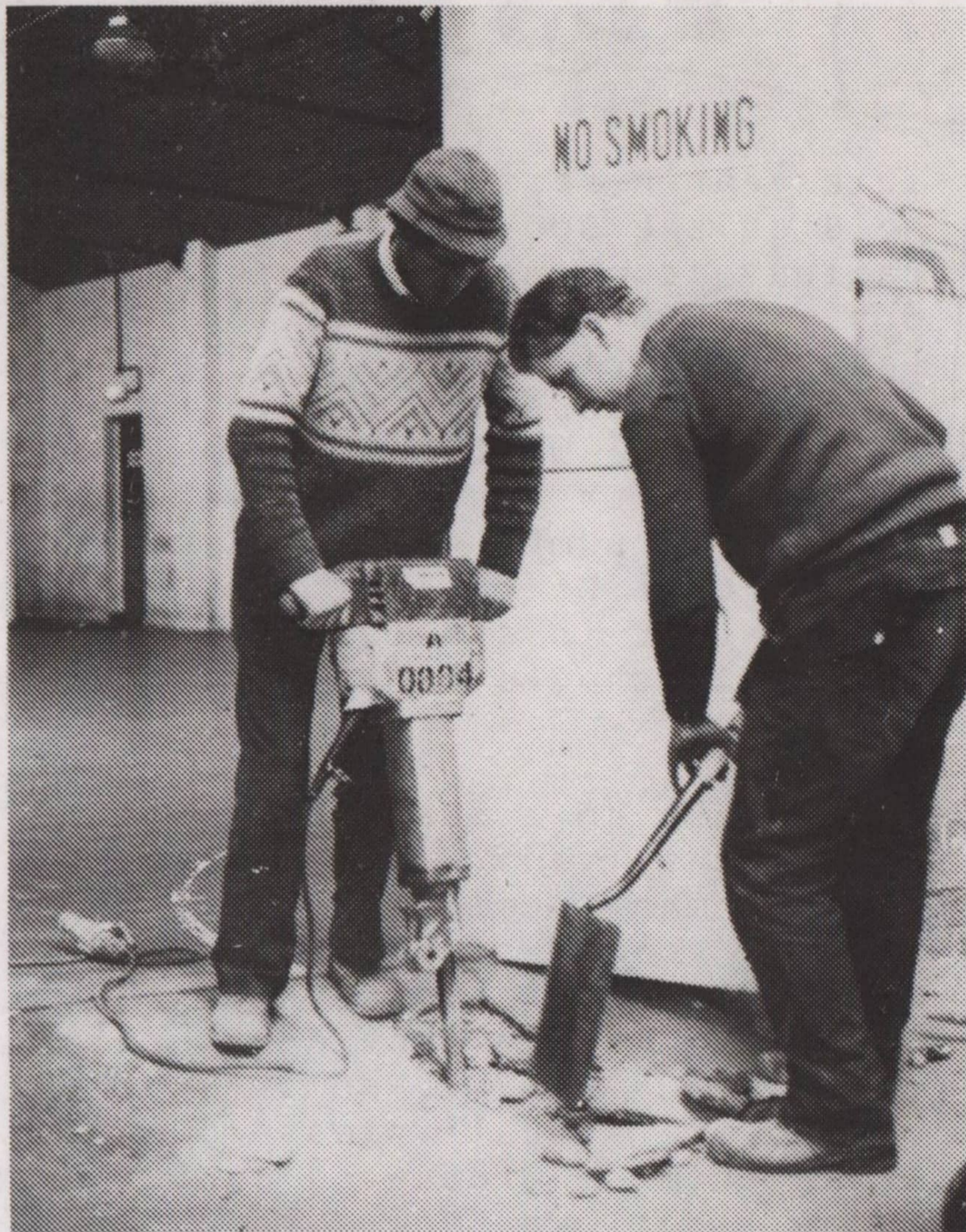
Conversion work begins!
