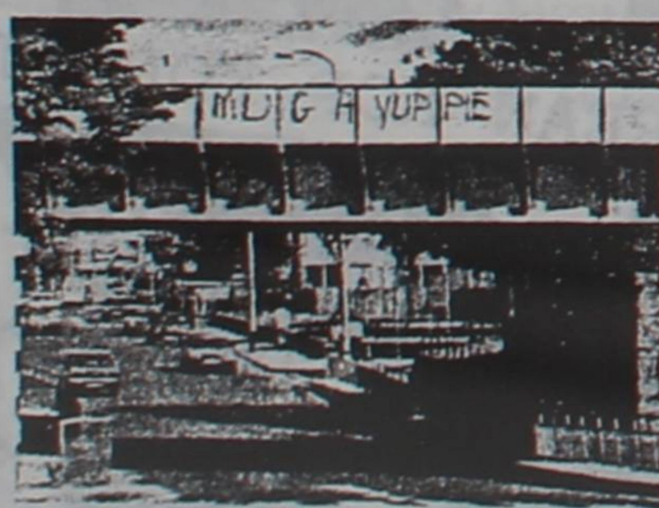
Grove Road railway bridge, Bow, E. London.
