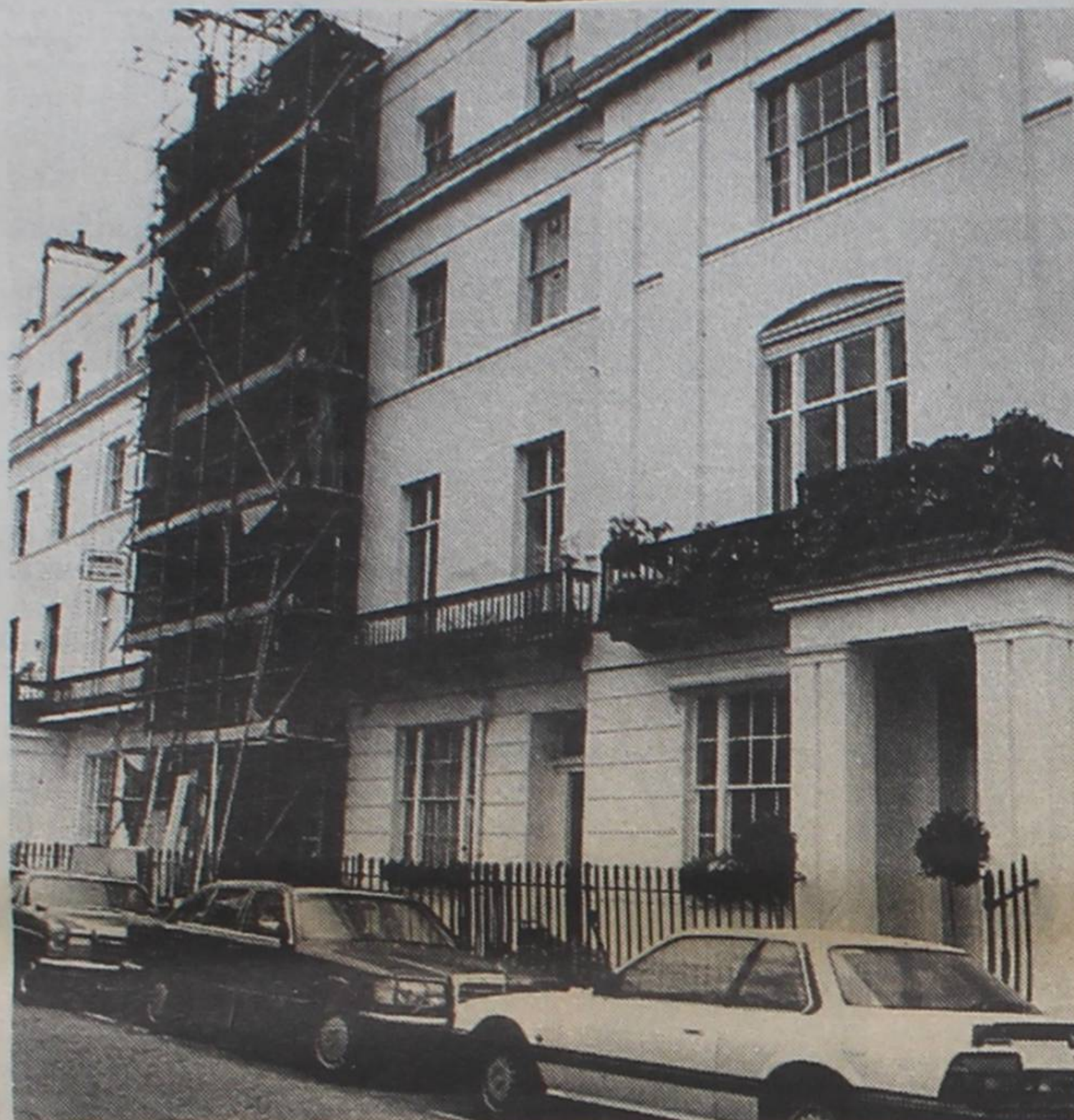
MAGGIES NEW HOUSE (THE ONE WITH SCAFFOLDING ON IT)
