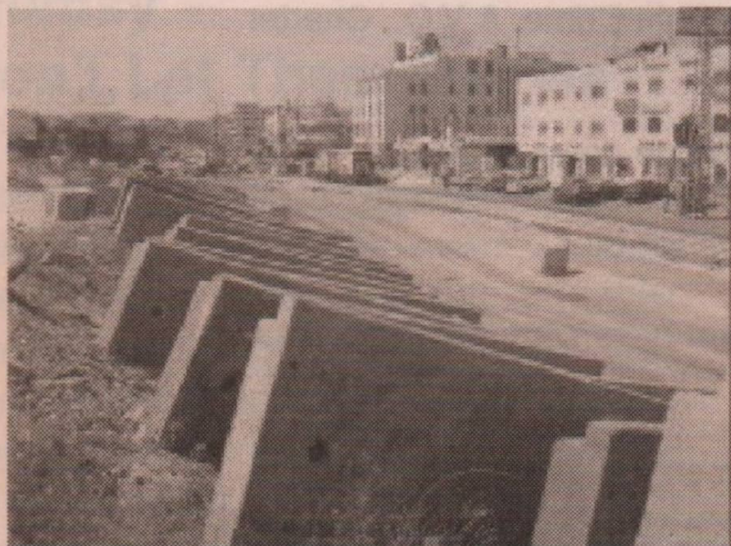
Construction of the Wall in Ar-Ram
