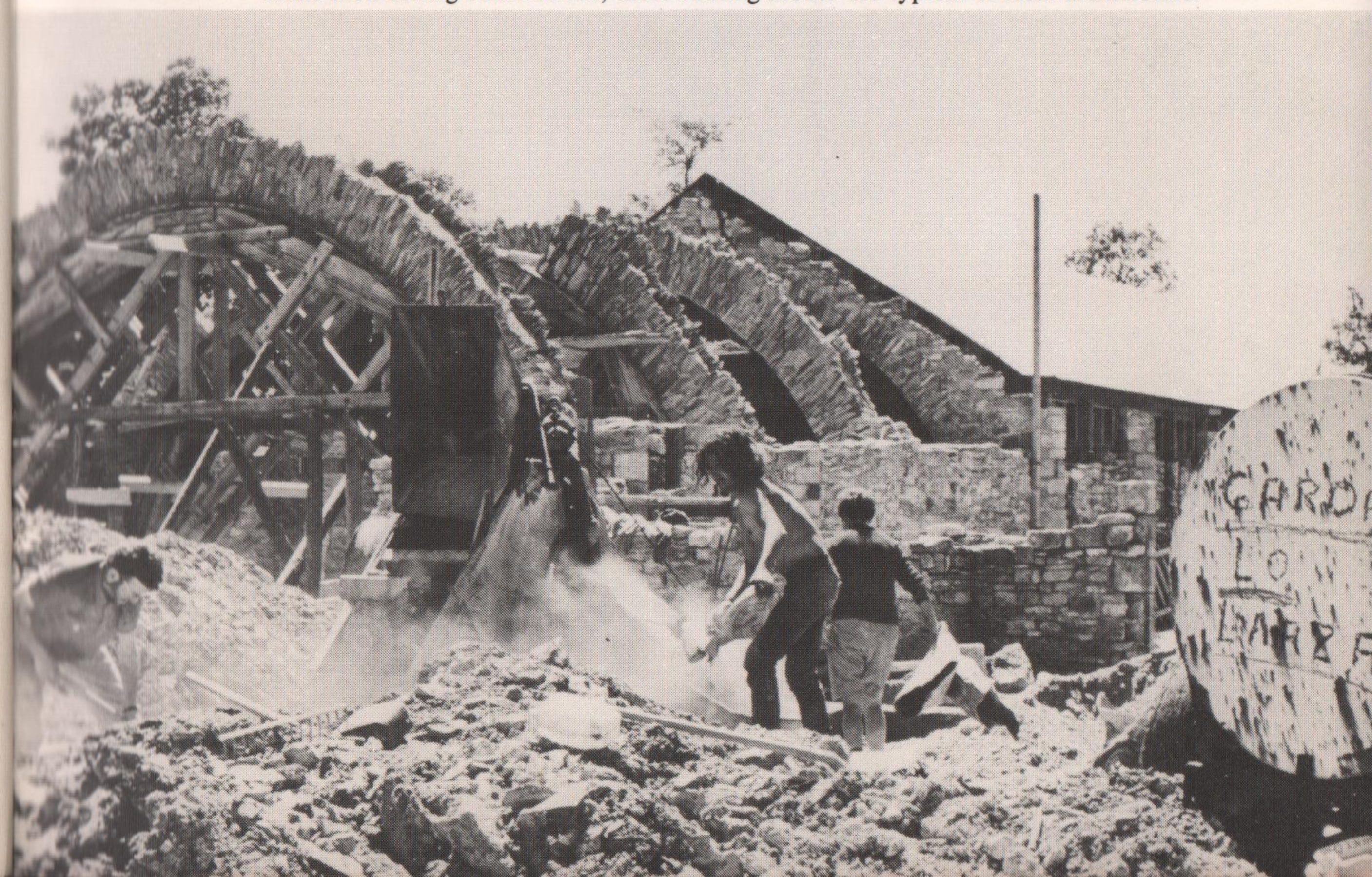
Below: Voluntary workers building the 'bergerie' or sheep farm at La Blaqui re without official permit in June 1974. The wooden structure forms the temporary centre support for the stone arch during construction; these roofing arches are typical of local architecture.
