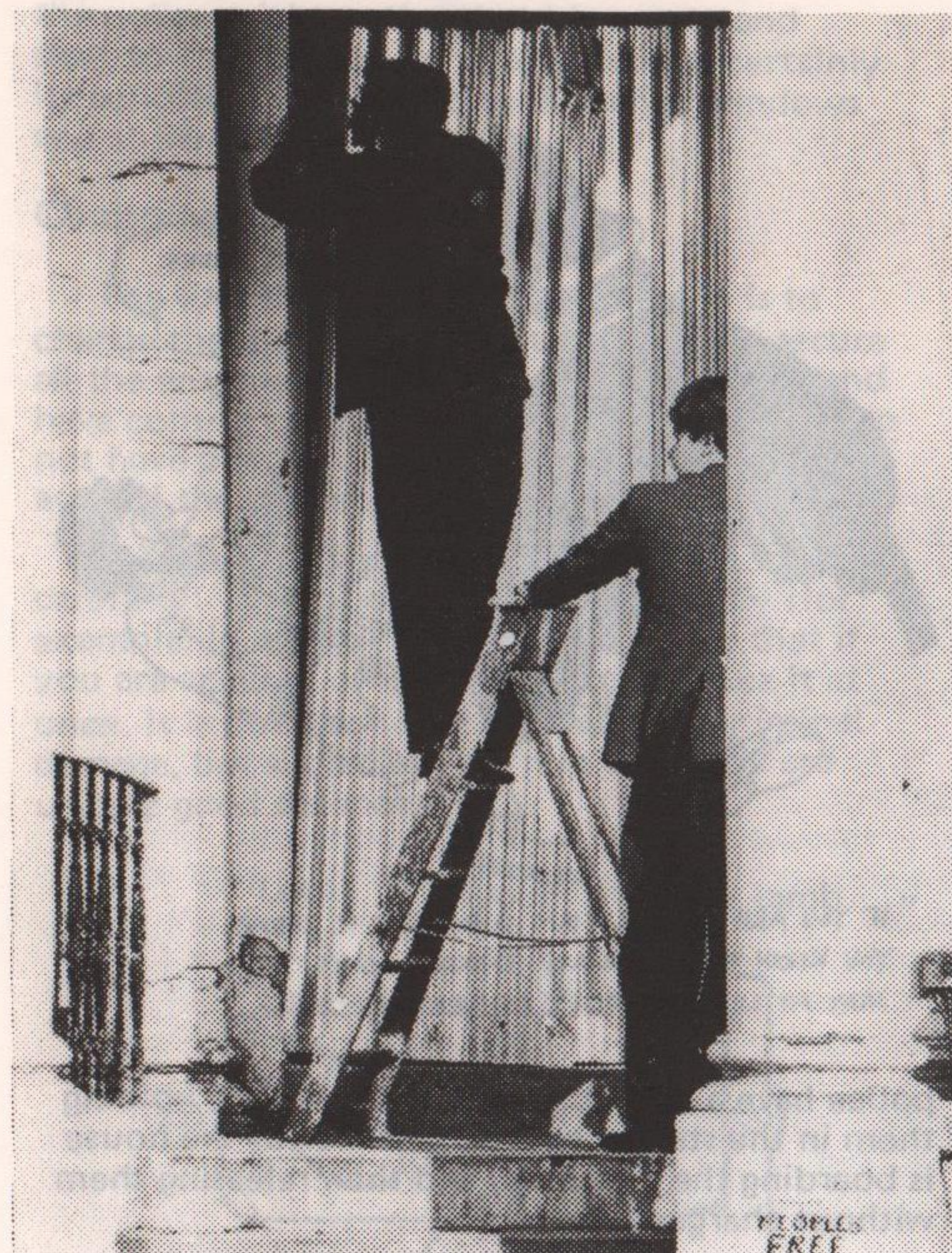
Removing corrugated iron
