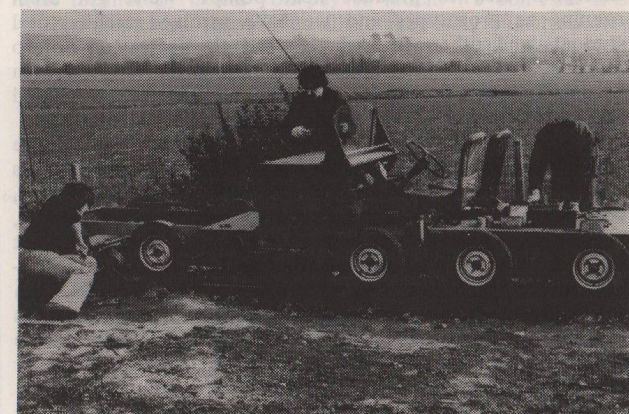
The first prototype of the Road/Rail Vehicle — one of the Lucas Combine's socially useful products (photo: CAITS)
